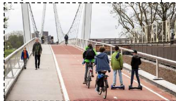
Pedestrian Lane and Bicycle Lane
