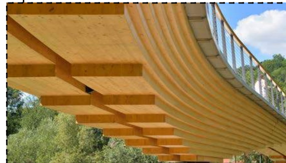
Mass Timber Superstructure
